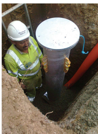
A2032 Worthing-Installation of Orion Socket
